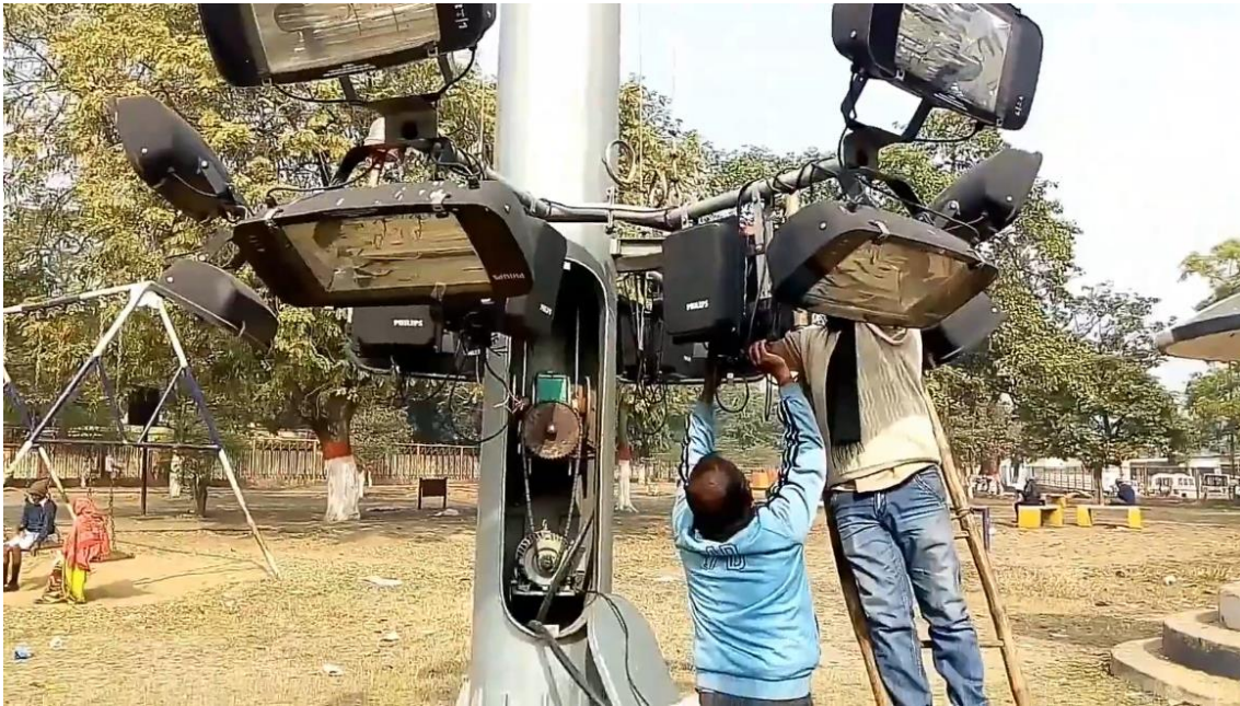
Figura 8. High mast lowering system
